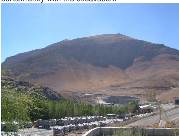
The Ghomrud water tunnel, downstream portal.
