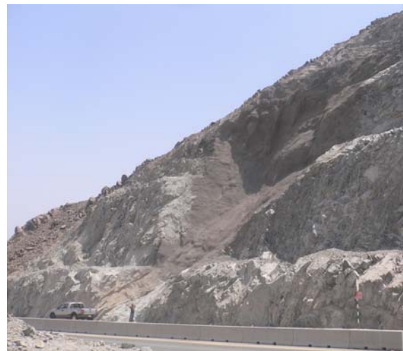
Dry sprayed concrete with MEYCO ® FIB SP540 used for slope stabilisation
