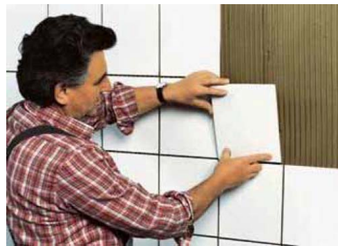
Reliable laying of tiles in the thin-bed method with Mastertile 11
