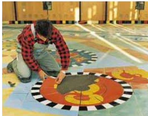
Secure laying of tiles with Mastertile 21
