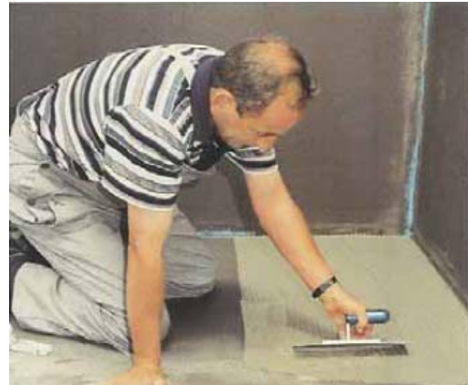
Tile adhesives modified with PCI Lastoflex HT reduce elongations of the substrate and compensate tensions caused by variations in temperature.
