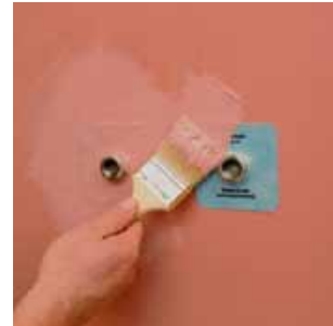
4. Place PCI Pecitape 10x10 over the pipe connection protruding from the wall and cover with PCI Lastogum (red)
