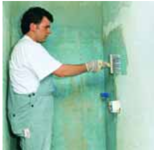
1. Priming: Prime absorbent mineral or gypsum-based substrates and plaster boards with PCI Gisogrund.
