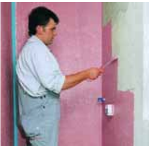
2. Apply undiluted PCI Lastogum (red) to the substrate as a first protective coating to cover its entire surface.
