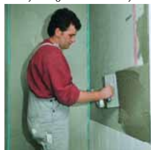
6. When the waterproofing PCI Lastogum has cured tiles can be laid.
