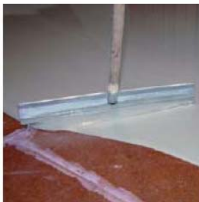
Spread to the required thickness with a suitable surface scraper
