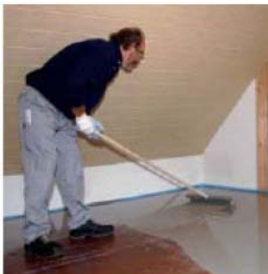
And de-aerated with a spiked roller.
