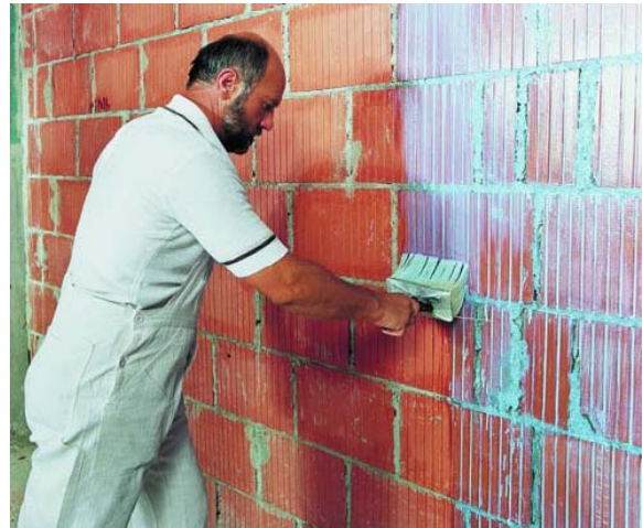
PCI Primer Gisogrund helps improve adhesion of plaster and lime plastering to brickwork.
